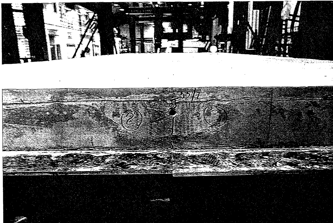
Fig. 8. A crack in the middle of the concrete tie beam, between the slab unit no 2 and 3.
